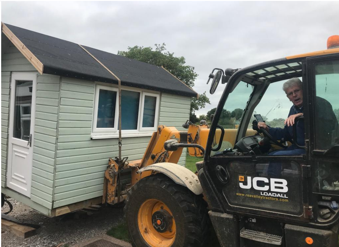
John moving the shed from the Vicarage garden to end of the lock up/hall.
